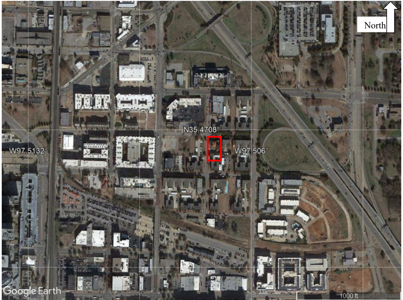
The Big Picture: Aerial (Google Earth 2018)
